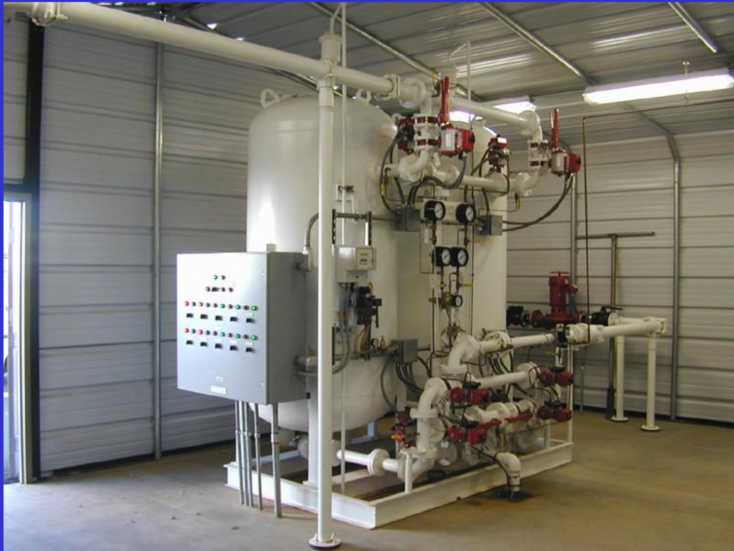
Skid-mounted vertically oriented Ferrosand filtration system (photo courtesy of Hungerford & Terry, Inc.)
